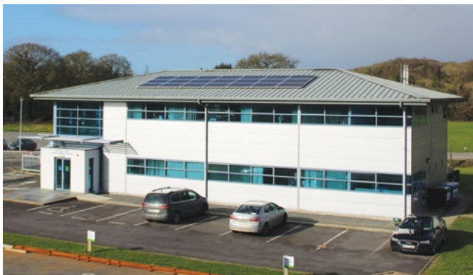
Installation of solar panels at Ballineen
